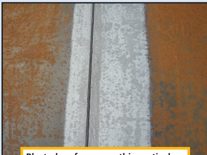
Blasted surface area, this particular model is fast and efficient in the removal of coatings, paint and rust.
