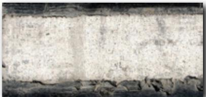
Utilize the milling cutter for removing thick and soft materials such as: mastic, thermo-plastic, waterproofing membranes, cold plastic coatings, glues, etc... It leaves the surface smooth and ready for preparation. Often used to remove bulk of material prior to a carbide tip cutter.
