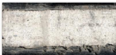
Utilize the milling cutter for removing thick and soft materials such as: mastic, thermo-plastic, waterproofing membranes, cold plastic coatings, glues, etc... The milling cutter leaves the surface smooth and ready for preparation.
